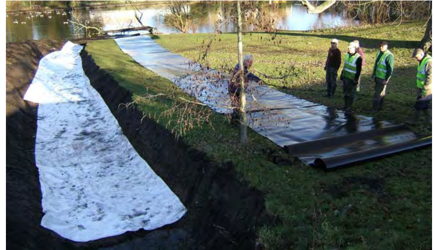
The protective blanket has been laid and the troops are ready with the butyl liner.
